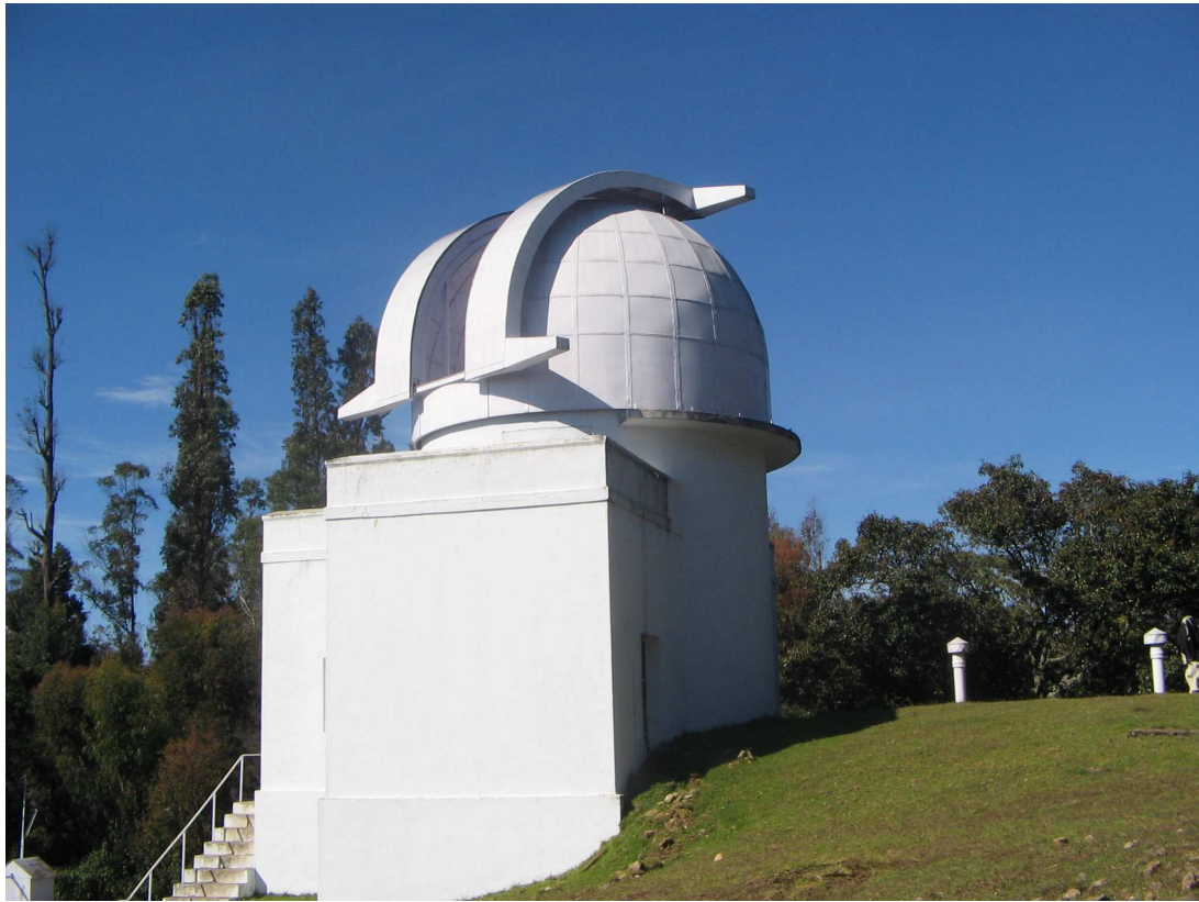
Figure 1.3: Tunnel telescope at the Kodaikanal Observatory. The tower contains a coelostat and a spectrograph, which is located in a 60-meter-long tunnel. The sunlight is directed by a flat mirror into the tunnel, which can be seen here as a grass-covered hill on the left with two cylindrical pipes used for the ventilation of the tunnel.
