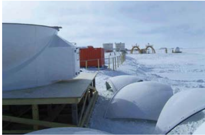
Fig. 6: During the erection of the ICE-T dome. The Concordia station is visible in the back.
