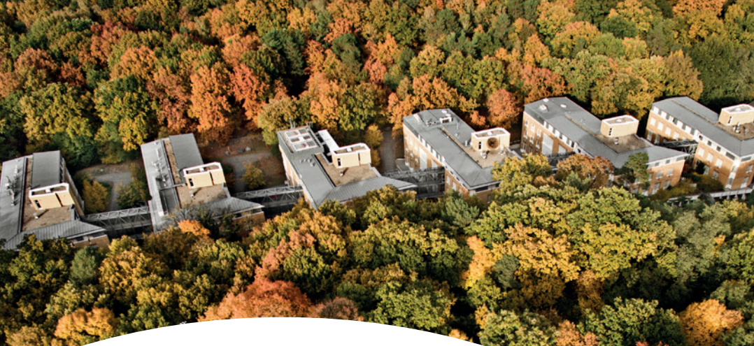
Aerial photograph of the GFZ buildings B-G, photo: JokeAir
