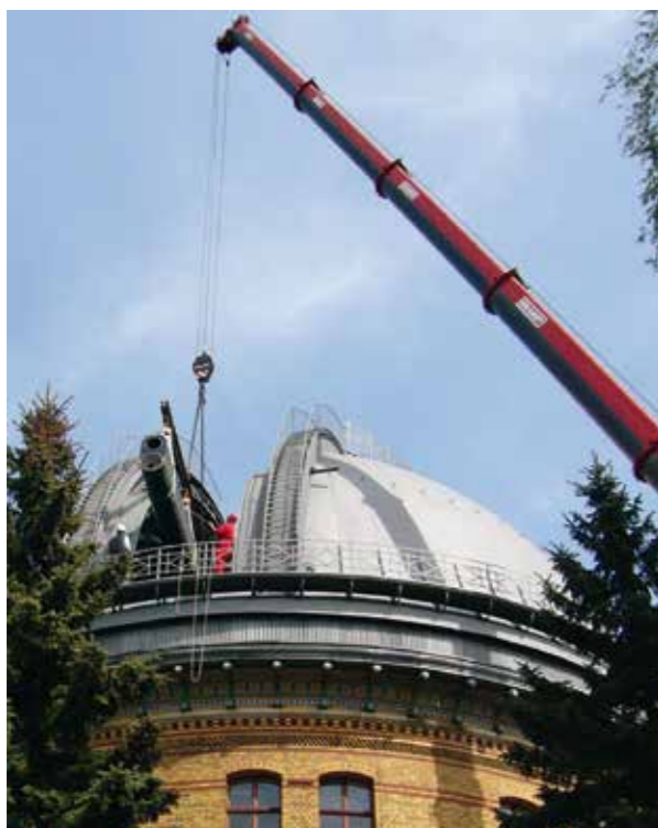
Disassembly of the refractor for restoration.
