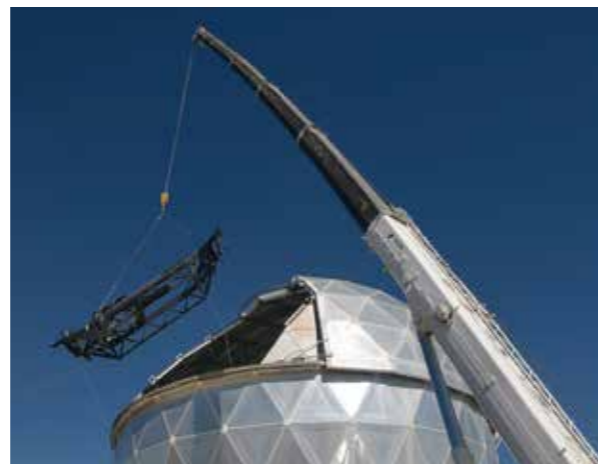
Fig. 3: Upgrade of the Hobby-Eberly Telescope at McDonald Observatory in Texas – the destination for the VIRUS instrument for the Dark Energy Experiment. (image: McDonald Observatory).
