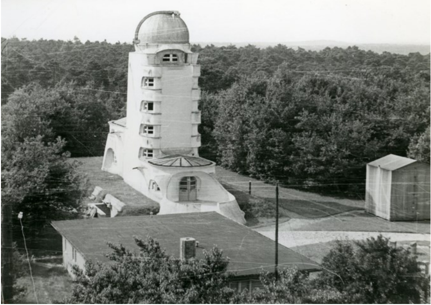
Fig. 31 Einstein Tower with Bosch barrack (foreground) and shelter (righthand) for expedition material. Source: ABBAW.
